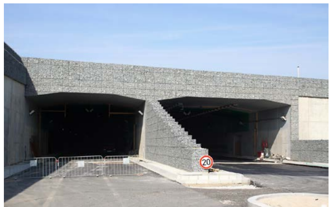
Figure 11 – Eastern portal of the Tunnel complex Blanka (Bubeneč)
