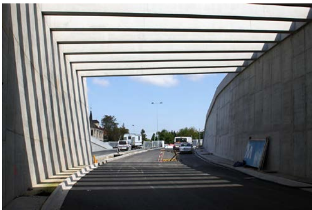
Figure 10 – U Vorlíků intersection, ramp 1 (Dejvice) – view from the portal
