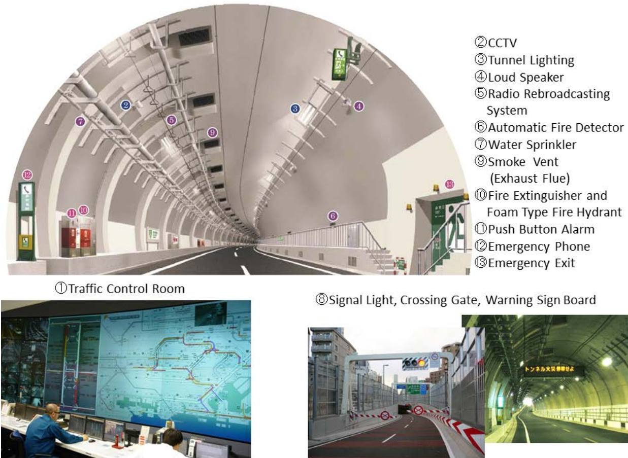
Figure 4 – main safety and operation equipment in Yamate Tunnel
