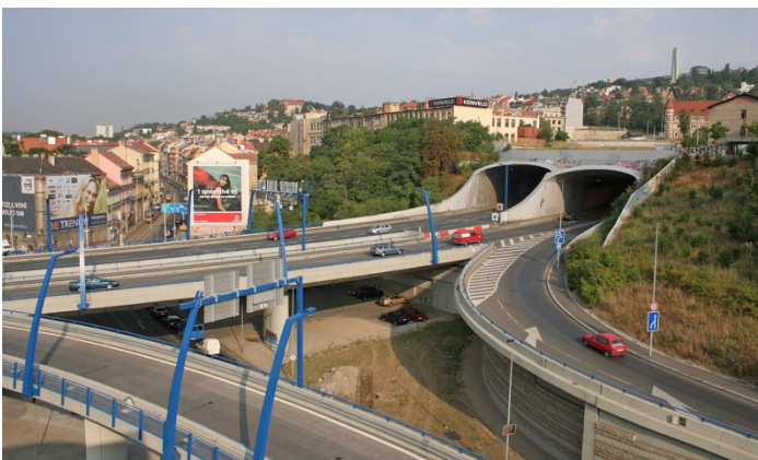
Figure 6 – Southern portals of Strahov tunnel and the bridge leading to Mrázovka tunnel
