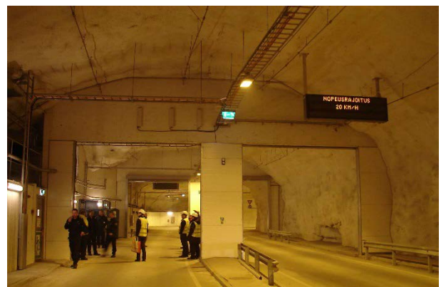
Figure 9 – curtain and FFFS at the bottom of a shaft
