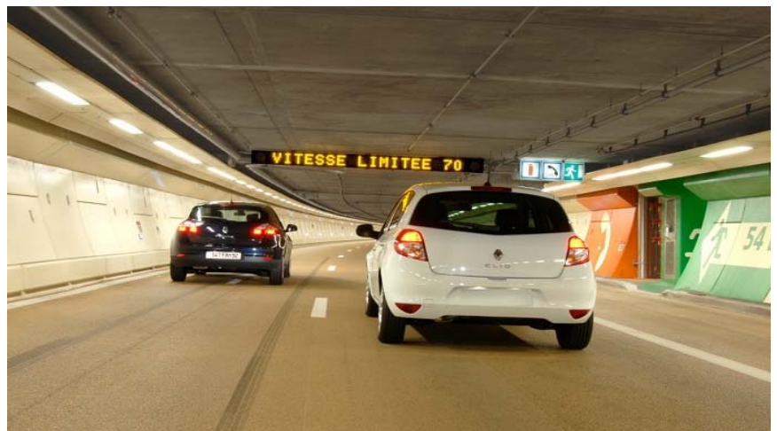
Figure 7 – view of specific VMS
