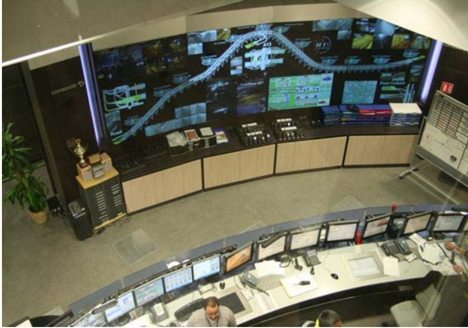
Figure 9 – view of the Duplex Tunnel's central control centre
