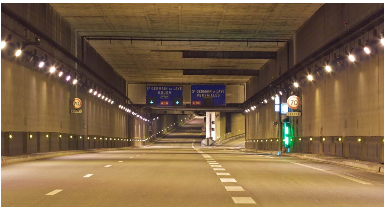
Figure 4 - motorways interchange A 14 / A 86 (AM/CETU)
