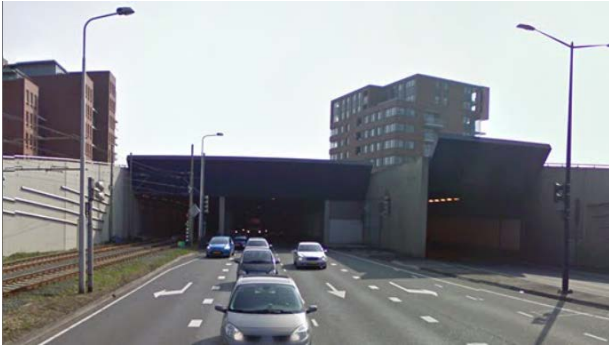
Figure 2: Vliet Tunnel road and rail tubes
