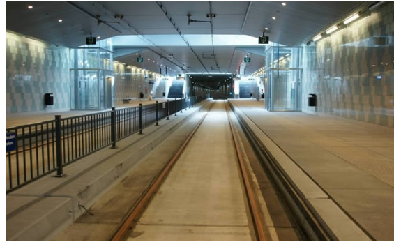
Figure 3: Underground rail station in the Vliet Tunnel
