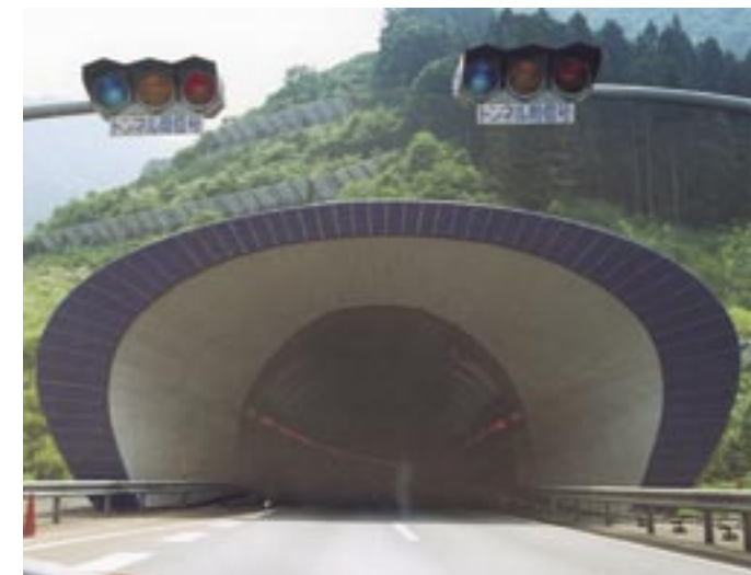
Figure 26: Portal of Kanetsu tunnel in Japan
