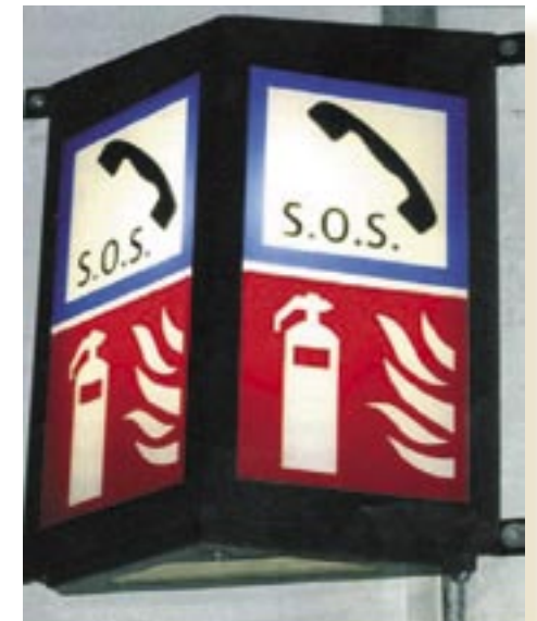
Figure 38: Sign to indicate fire extinguishers as prescribed in Dutch guidelines
