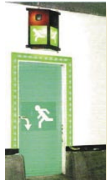
Figure 44: Example of emergency exit with LED-frame (lighting only in case of emergency), permanently illuminated pictogram for emergency exit and sound beacon above the exit (The Netherlands)
