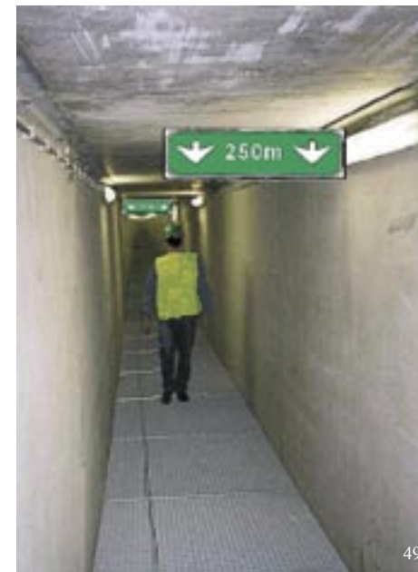
Figure 49: Panel mounted on the ceiling of escape galleries between tunnel tubes to indicate direction and distance to the open area
