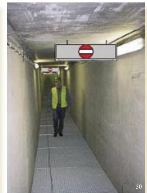
Figure 49: Panel mounted on the ceiling of escape galleries between tunnel tubes to indicate direction and distance to the open area
